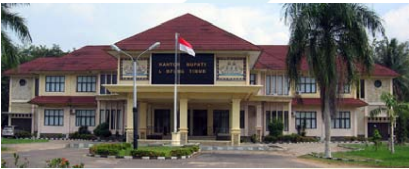
East Lampung, Regent's Office
